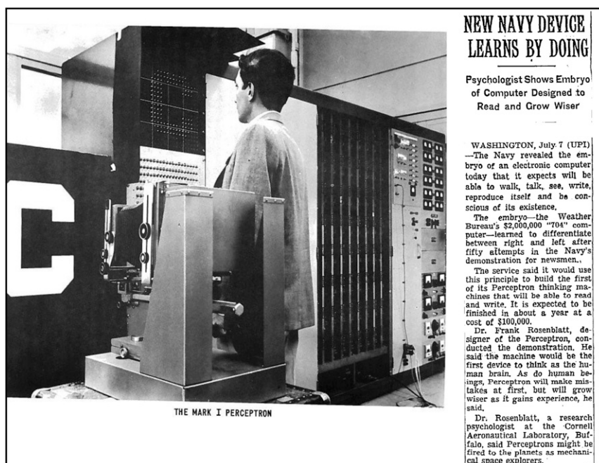
Fig. 3. Early perceptrons were large-scale analog systems (3). (Left) An analog perceptron computer receiving a visual input. The racks contained potentiometers driven by motors whose resistance was controlled by the perceptron learning algorithm. (Right) Article in the New York Times , July 8, 1958, from a UPI wire report. The perceptron machine was expected to cost $100,000 on completion in 1959, or around $1 million in today's dollars; the IBM 704 computer that cost $2 million in 1958, or $20 million in today's dollars, could perform 12,000 multiplies per second, which was blazingly fast at the time. The much less expensive Samsung Galaxy S6 phone, which can perform 34 billion operations per second, is more than a million times faster. Reprinted from ref. 5.
